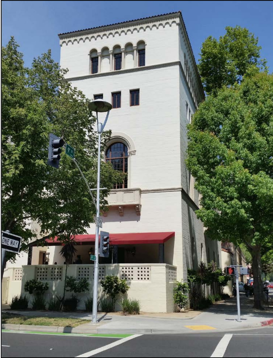
Photograph 2 of 4 - East wing of the Sutter Club, view northwest from Capital Mall and 9th Street intersection.
