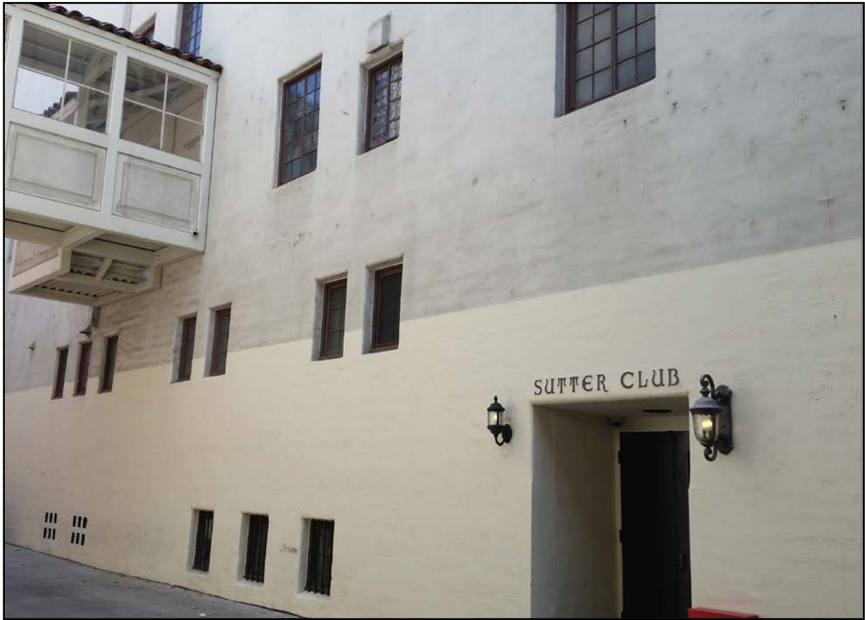
Photograph 4 of 4 – North elevation, view southeast from the alley.
